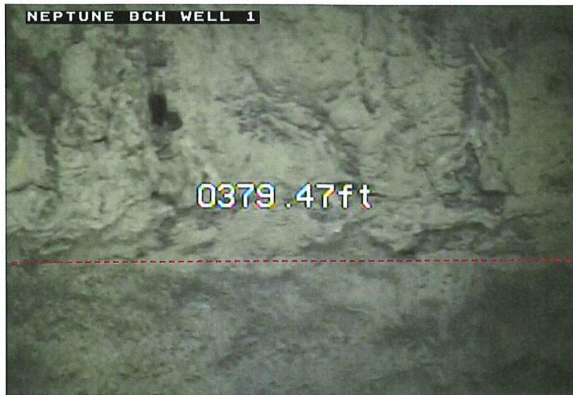
Photograph 6 -Bottom of Casing Side View
