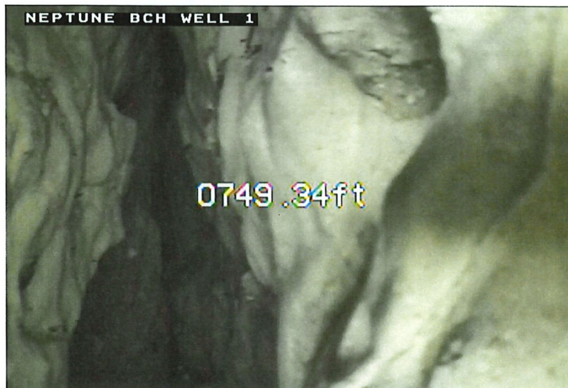
Photograph 7 - Water-Bearing Fractures and Voids in Open Hole
