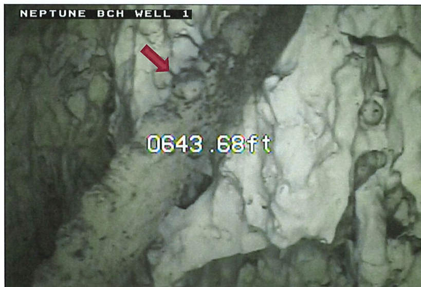
Photograph 5 - Metal Strap/Rod Observed in Well
