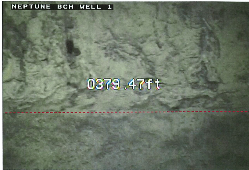
Photograph 6 -Bottom of Casing Side View
