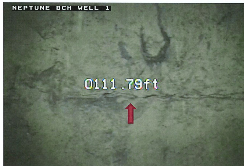
Photograph 2 - Typical Casing Joint at 111 feet
