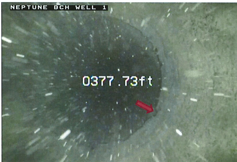
Photograph 4 - Bottom of Casing Looking Down
