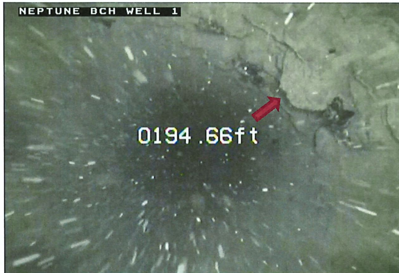
Photograph 3 - Casing Incrustations (Looking Down in to Well)
