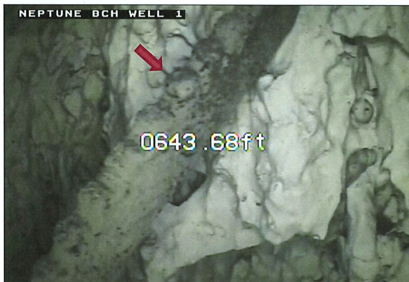
Photograph 5 - Metal Strap/Rod Observed in Well
