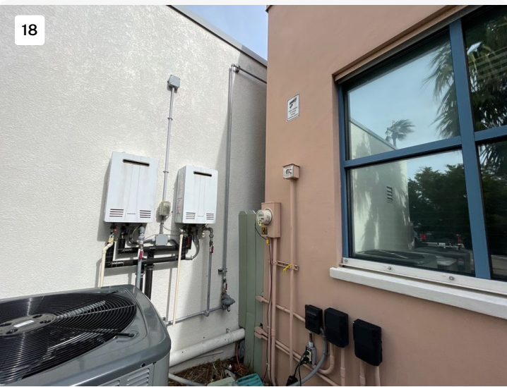
tight space between buildings on north side.
