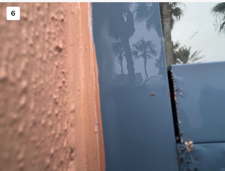
Water test showing water intrusion at windows around window seals and mullion entry points
