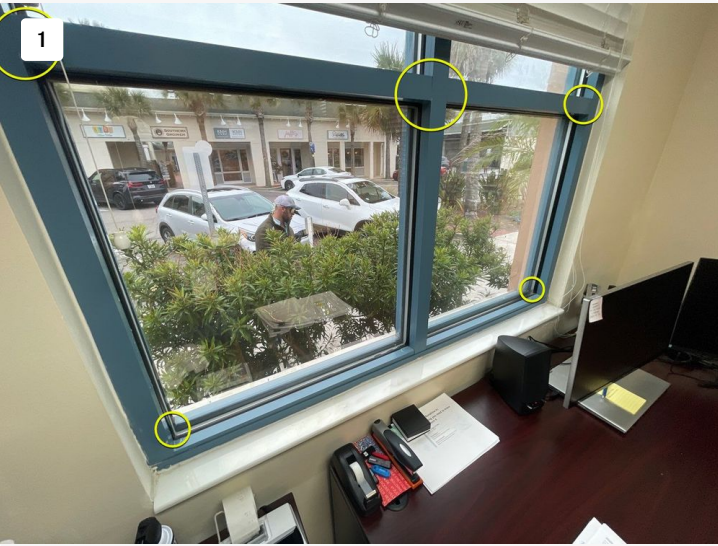
Water intrusion points illustrated
