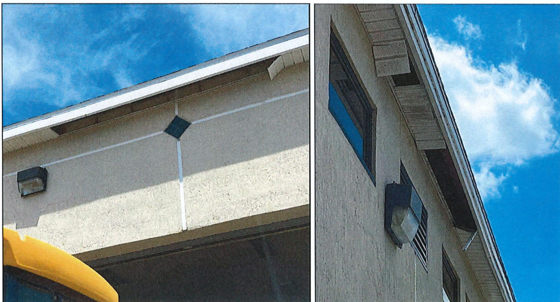
Typical soffit damage
