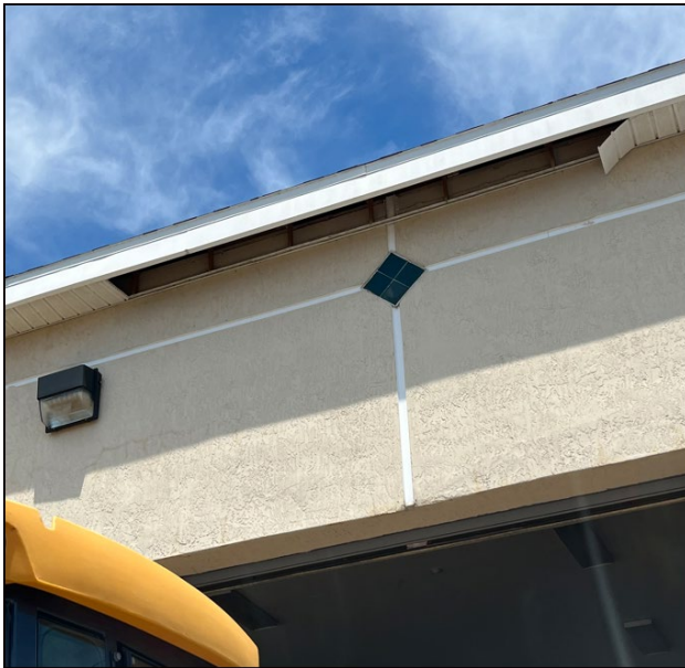
Typical soffit damage
