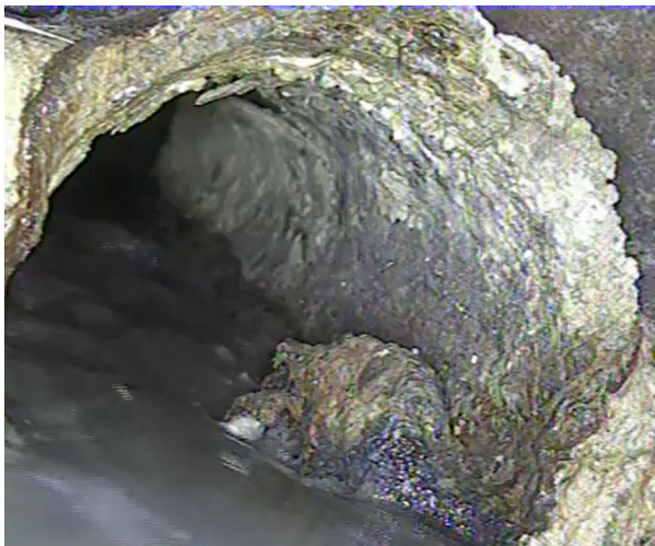
Pipe at Manhole
