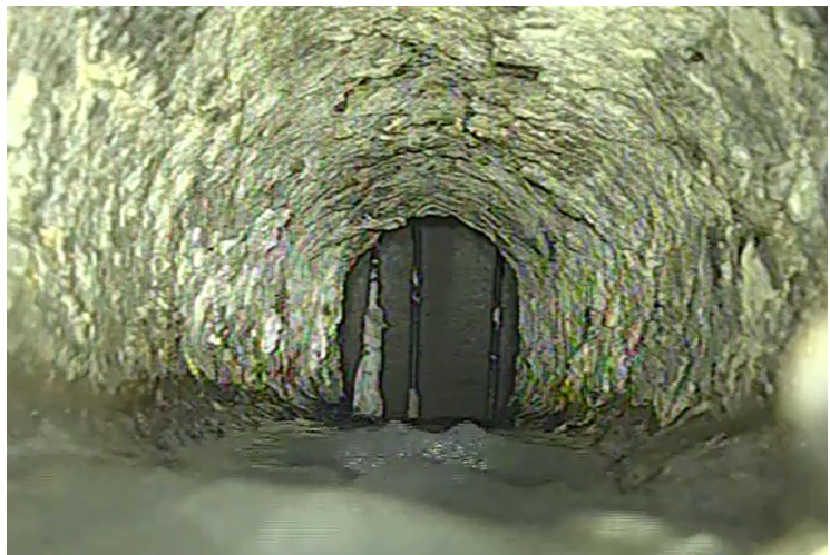
Approaching Pump Station Wet Well
