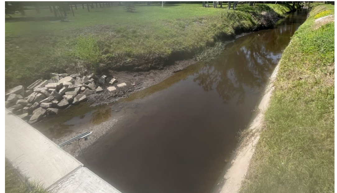
Example undermining of ditch bank at Basil Park
