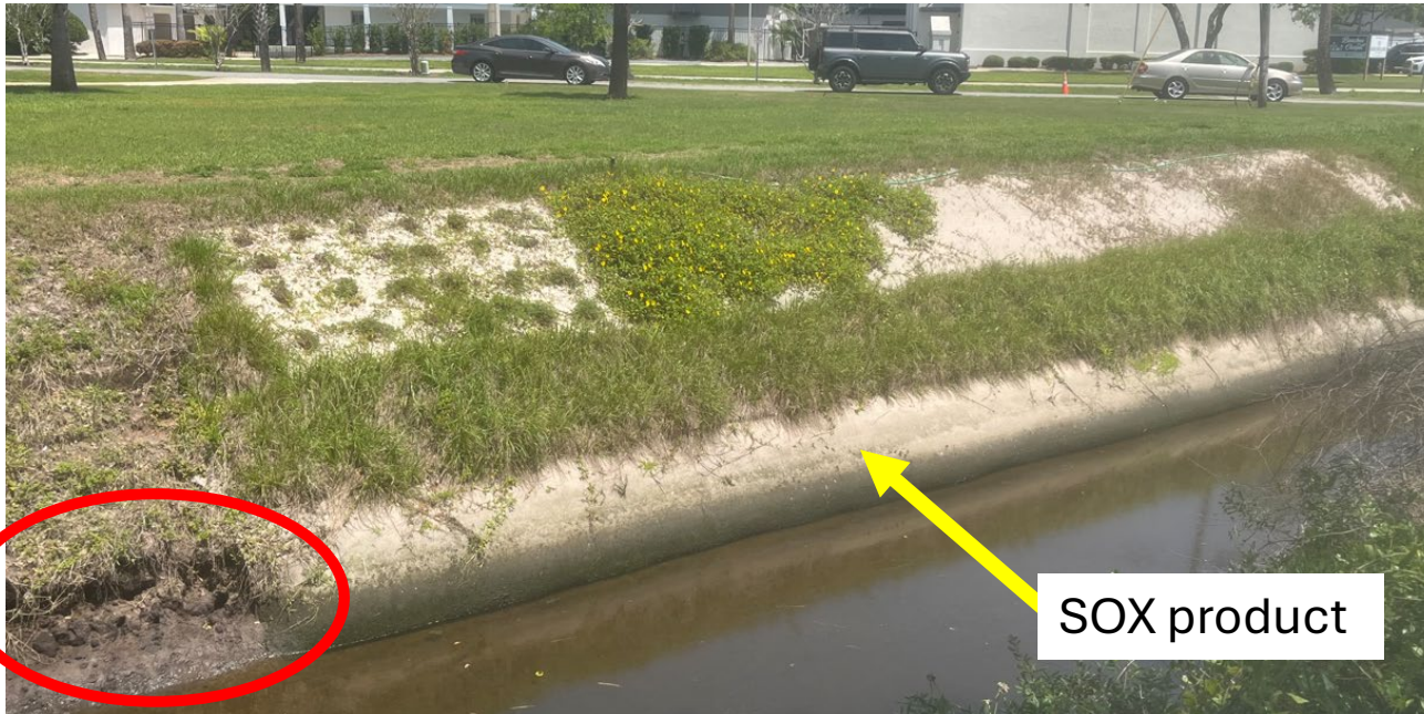
Example undermining of ditch bank at Basil Park
