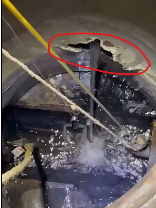
Infiltration at Failed Manhole Bench
