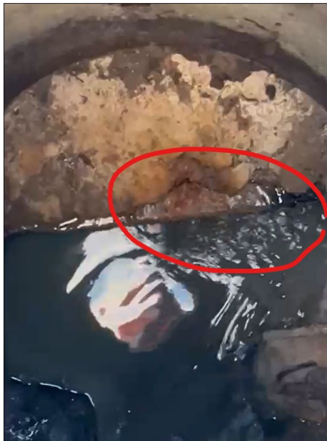
Infiltration at Failed Manhole Bench
