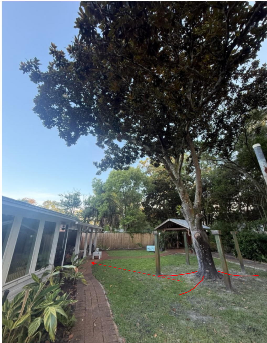
Water shedding away from tree due to raised elevation causing flooding to back patio and intrusion into garage.
