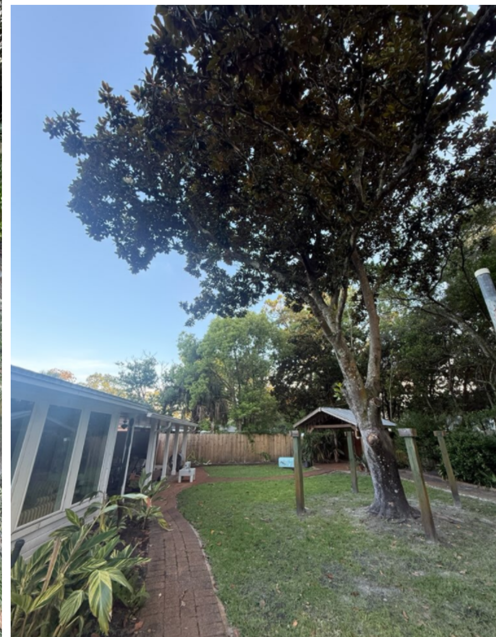
Tree leaning over house. Tree canopy coverage over 50% of back yard, creating concern of falling limbs or debris where kids can play.
