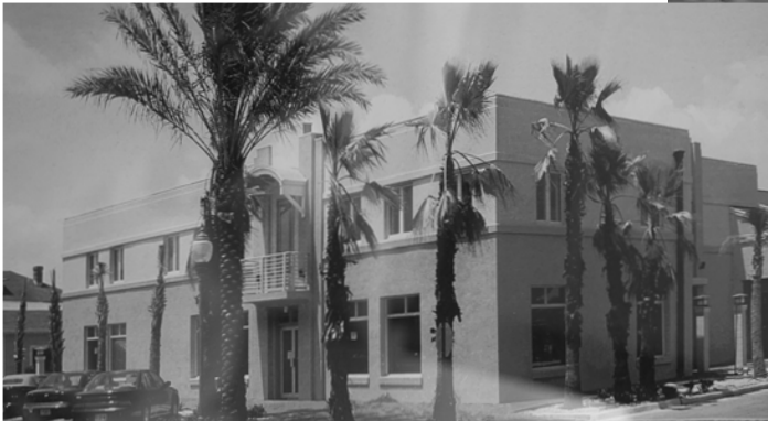
Adaptive Reuse of 200 First Street: Before & After
