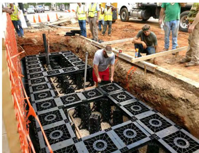
Figure 4.86: Tree wells with Soil Cells
