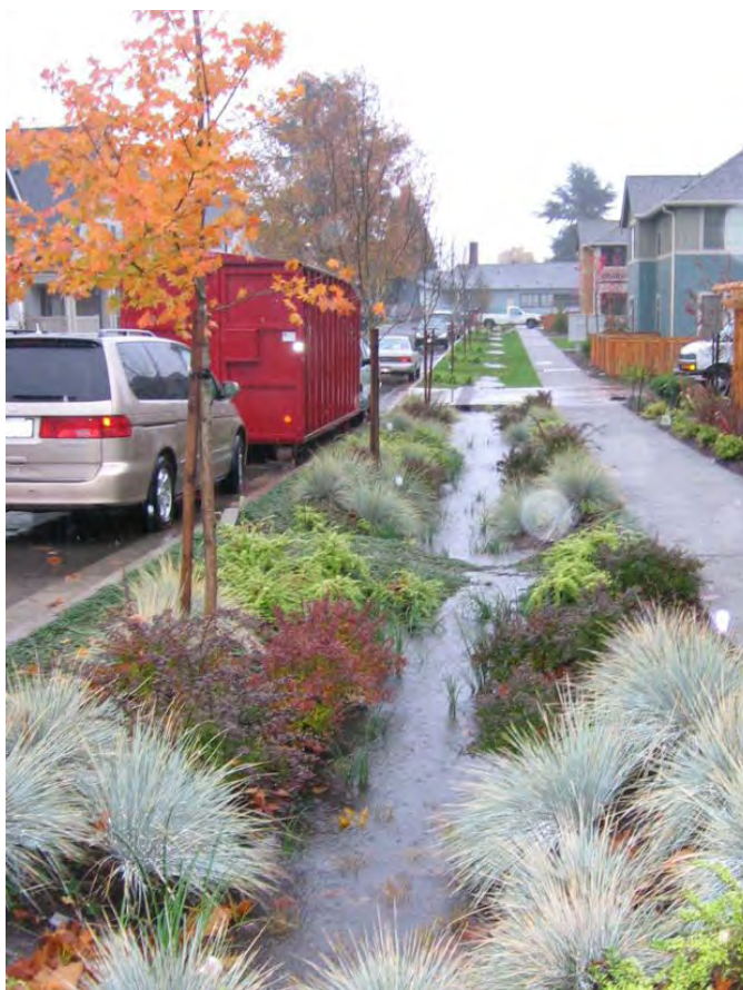
Figure 4.88: Bioswale filters stormwater
