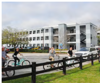
Sky Enterprises Office Building
