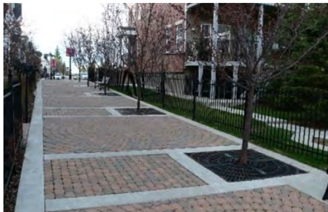
Figure 4.87: Pervious pavers with tree wells
