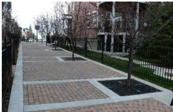
Figure 4.65: Pervious pavers with tree wells
