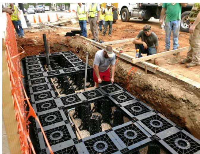
Figure 4.64: Tree wells with Soil Cells
